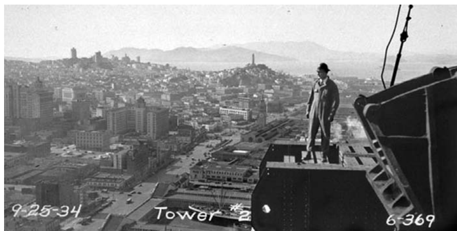
San Francisco-Oakland Bay Bridge w 1934 r. Fot: Wikipedia.
